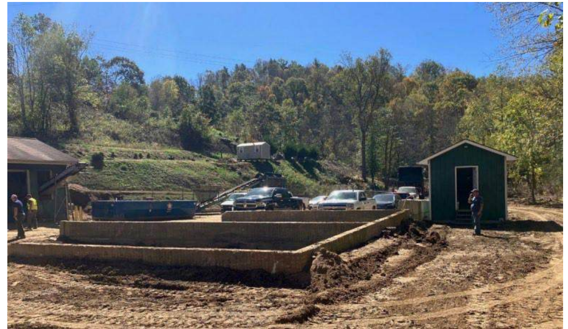
Effluent sampling building and compost staging beds at Burnsville WWTP, 10/10/24
